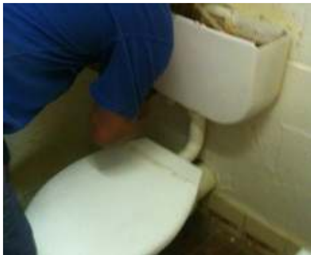
New Toilets, Shower Roses & yes Hot Water
